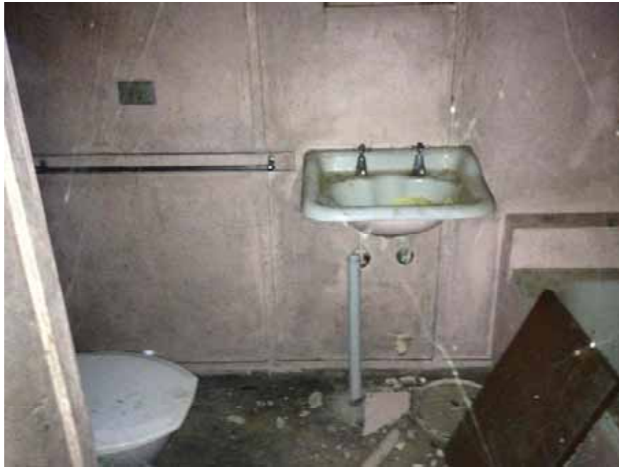
Photograph 31 – 65 Kowan Rd, Asbestos containing flat sheet bathroom wall linings
