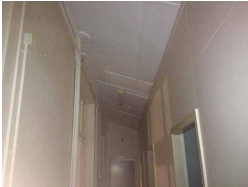
Photograph 23 – Building 12, Asbestos containing flat sheet ground floor ceiling lining
